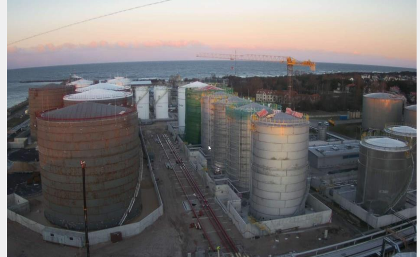
LFO 2 x 10 000 m 3 and 4 x 5 000 m 3 tanks installation - Installation of tanks wall plates and tank park concrete walls ongoing. 2x10 000m 3 tanks erected in full height. Hydrotesting completed. Ongoing with internal painting.
