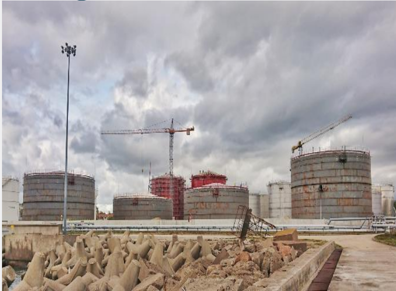
LFO 6 x 20 000 m 3 tanks installation - Installation of tanks wall plates and tank park concrete walls ongoing. Roofs of two tanks painted.
