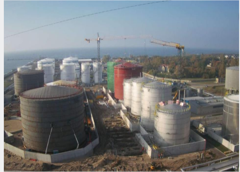
LFO 2 x 10 000 m 3 and 4 x 5 000 m 3 tanks installation - Installation of tanks wall plates and tank park concrete walls ongoing. 2x10 000m 3 tanks erected in full height. Hydrotesting completed. Ongoing with internal painting.
